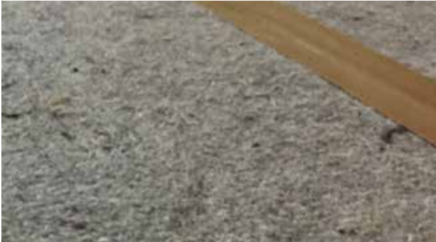
Figure 5: 7mm porous underlay
