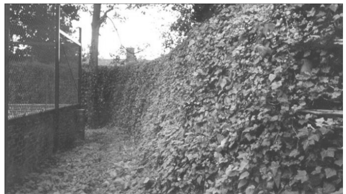
Figure 6(b): Retained soil bank with well established evergreen creeper (Weavewall Ltd).
