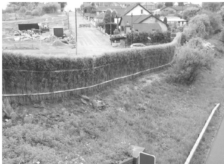
Figure 9: Growing woven willow fence with absorptive panel cores (ETS Ltd).
