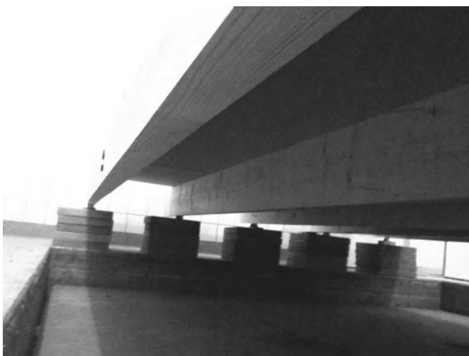
Figure 4: The beams and their supports, seen from below the floor.
