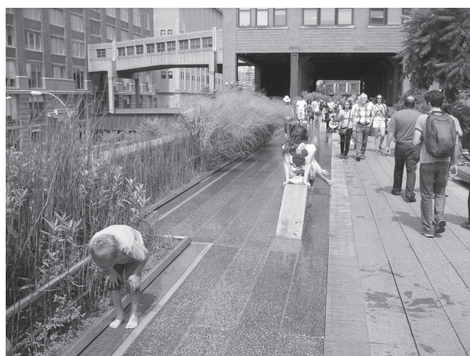
Figure 4: Section of the popular “High Line” in NYC cutting through the old industrial Meatpacking District showing laminar flow water feature and mixed wild grasses.
