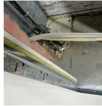
Figure 2: The traditional roof construction as seen in Figure 1 in practice. Condensation and black mould have formed in ceiling plenum of a school that is less than 2 years old. Furthermore, steel fixings have started to rust.
