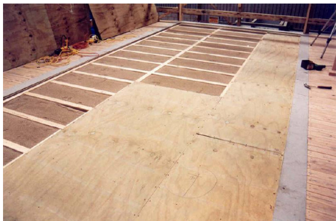
Figure 3. View of plywood flooring over 70x45mm battens laid on the flat with sand infill.
