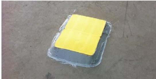
Figure 3. Typical packing under jack-up mounts
