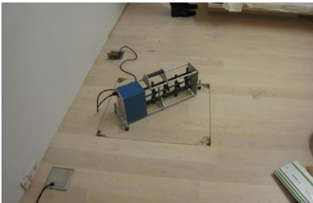
Photo 1. Floor test area with cuts & corners chiselled out
