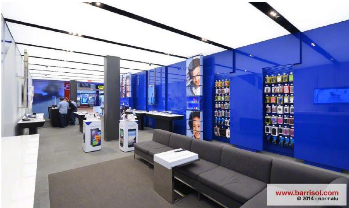
Figure 6: Sound absorptive, micro-perforated “daylight ceiling” modules.
