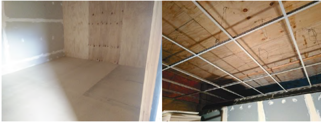
Figure 1: Overview of the CFN facility at the University of Canterbury
