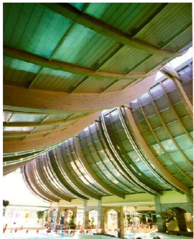
Figure 8: Sound absorptive, micro-perforated polycarbonate ceiling above a swimming pool.
