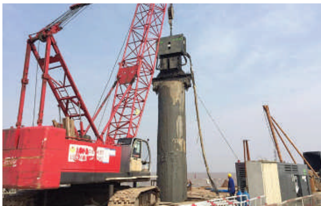
Figure 2: ICE 55NF vibro-piling rig
