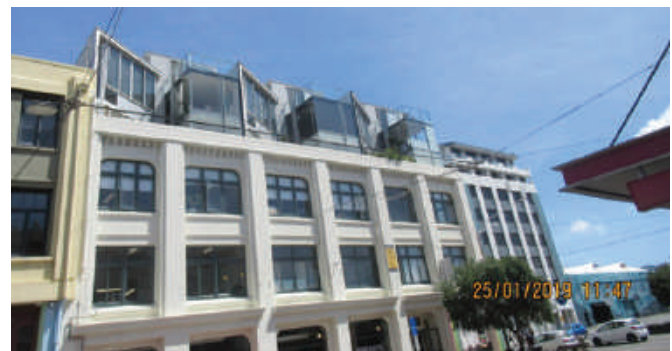
Photo 2: Measurements showed “internal noise levels” in these uninsulated apartments (glass wall façade) in the Courtenay Place area exceeded recommended levels for residential living when external levels met District Plan requirements
