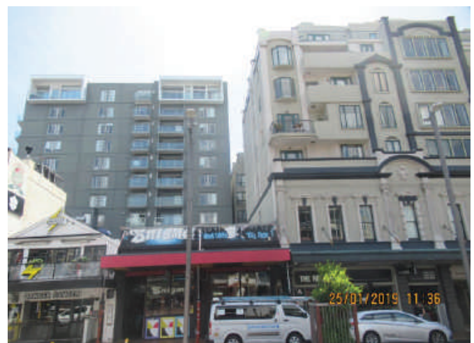
Photo 1: Recently constructed sound insulated apartments on the left and uninsulated apartments on the right bordering entertainment venues facing Courtney Place
