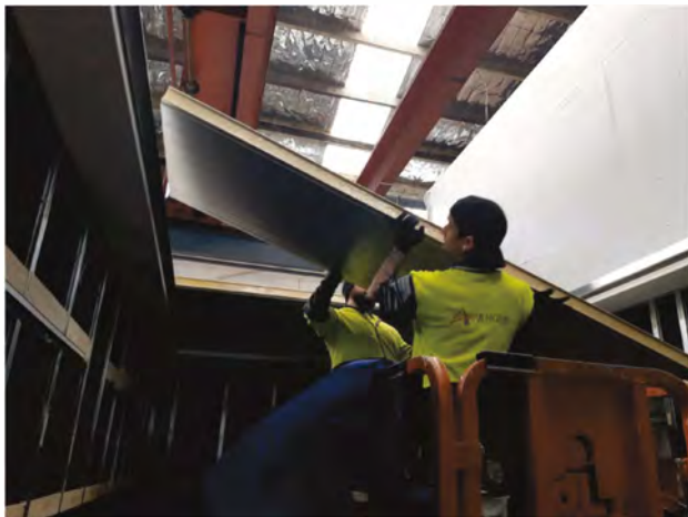
Figure 9 – Control room drop in ceiling being installed
